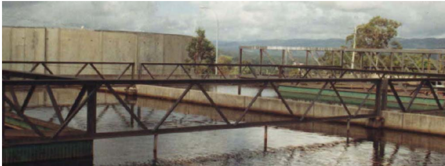
Figure 5.1 Truss structures spanning a clarifier in a water purification plant
