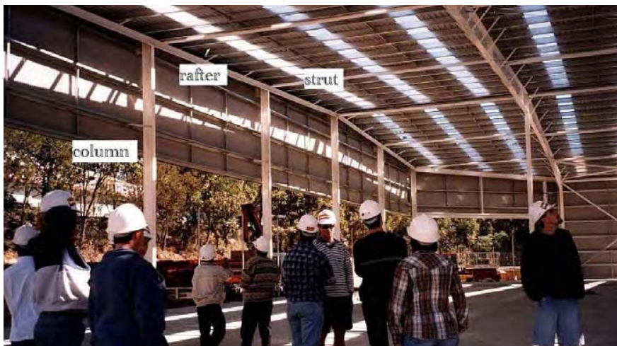
Figure 6.1 Compression Members include the Vertical Columns and the Horizontal Struts running across the picture
