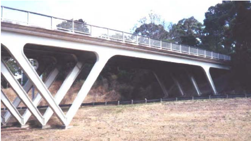
Figure1.4 Steel bridge structure supporting concrete deck, Adelaide Hills
