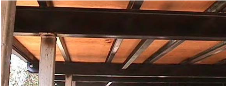
Figure 3.6 Typical Steel-Framed Floor Construction Showing Timber Sheeting and Steel Floor Joists, Bearers and Stumps
