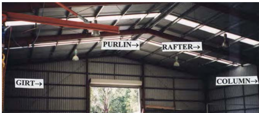
Figure 3.5 Roof Sheeting is Supported by Purlins, Rafters and Columns
